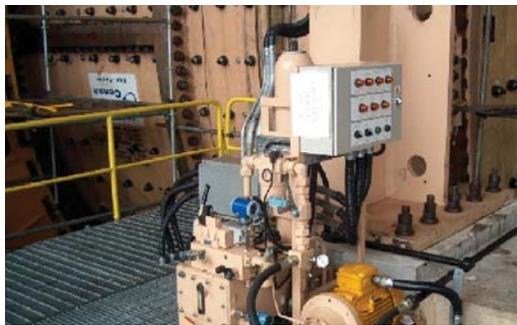
Figure 12: Hydraulic Powerpack
